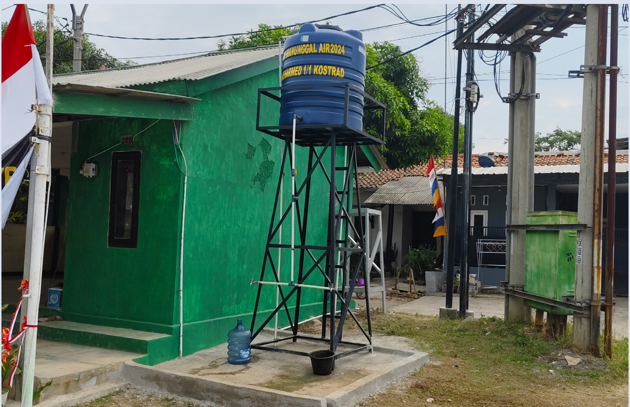
Sustainable water source: A water tank tower of 1,000 liter capacity in Campaka local community, Indonesia
