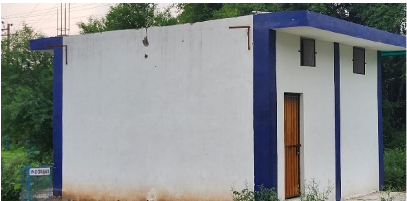
Newly constructed washrooms at the cremation ground in Manakpur, India
