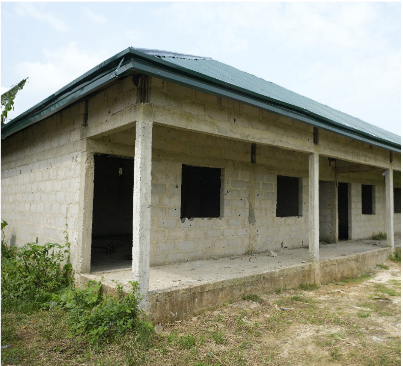
School under construction in the Onne community, Nigeria
