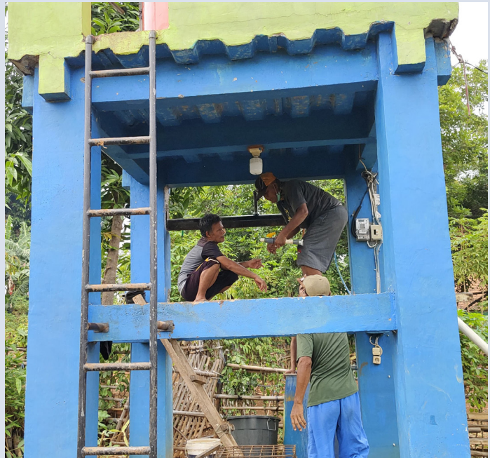
Borewell for sustainable groundwater access with 4,000 liter capacity in Kembangkuning Village, Indonesia
