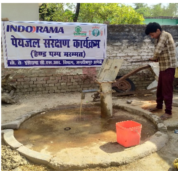
A man using a newly installed water handpump in Jagdishpur, India
